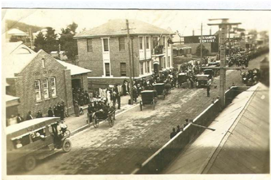
Figure 4 Wollombi Road in Bellbird with sandstone guttering in 1923 and also what could be a bitumen surface (Cessnock City Library 2023).
