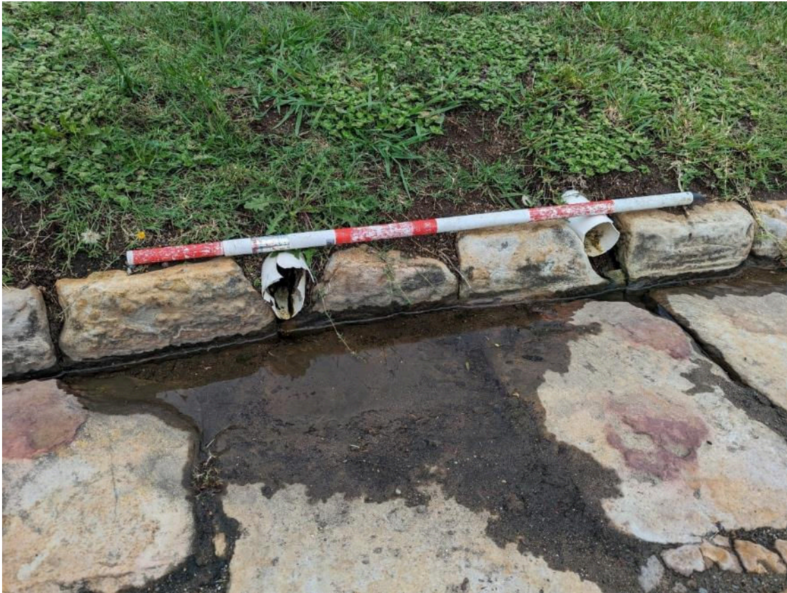
Figure 9. Sandstone kerb in the project area with cuts to accommodate drainage.
