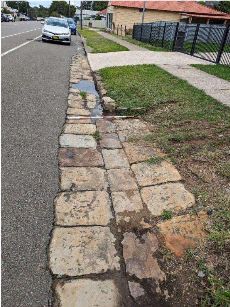
Photo 7 Standstone kerb and cut-in cement driveway
