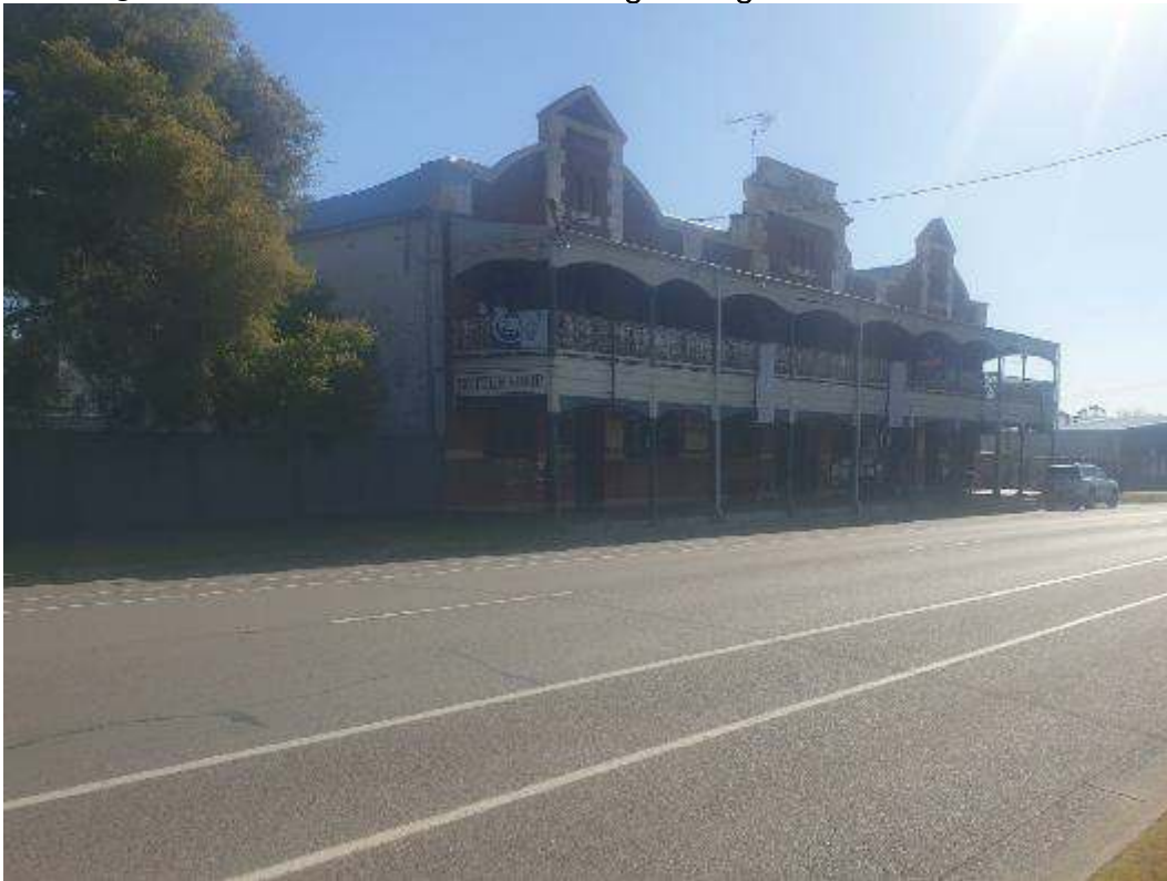
Figure 8 Bellbird hotel with sandstone guttering hard to see in this view
