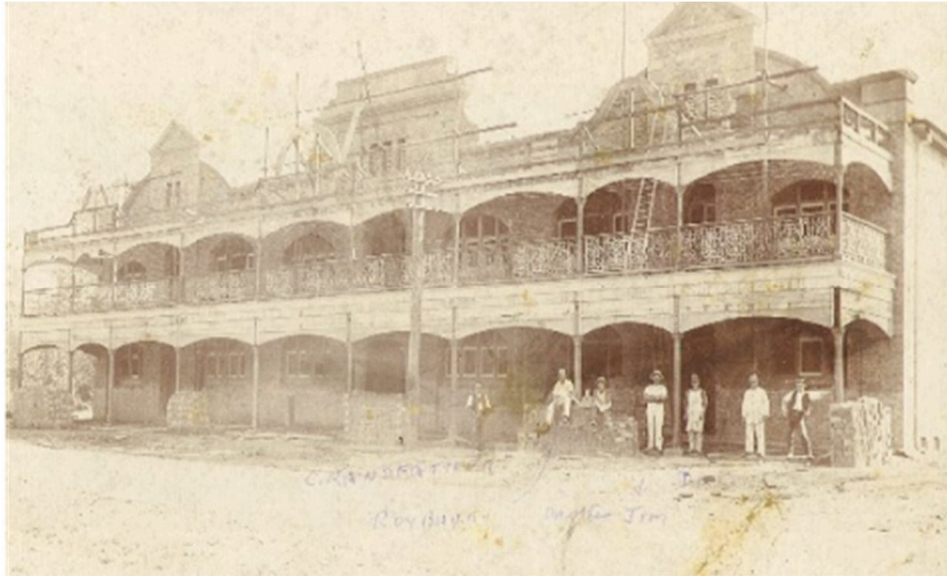
Figure 10. Bellbird Hotel during construction in 1914. Source: Cessnock City Library.
