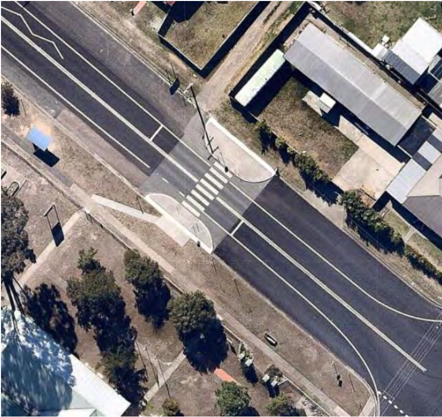
Figure 1 – Caledonia Street – Pedestrian Facility
