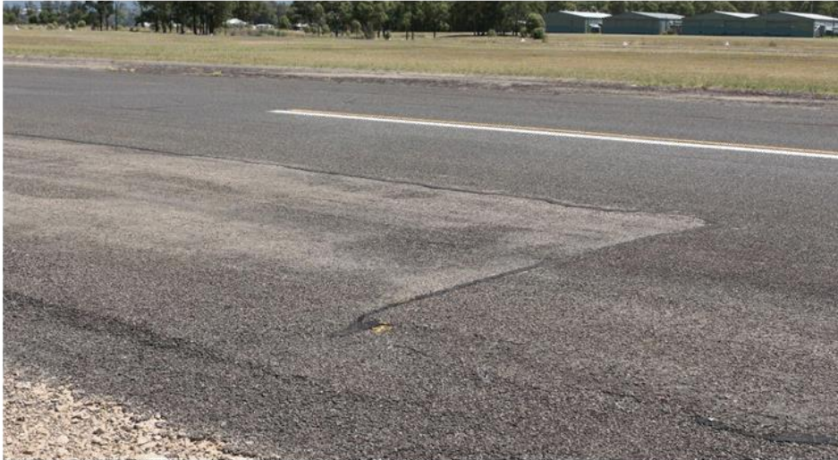
Figure 2-4 Degraded wearing course and uneven patches
