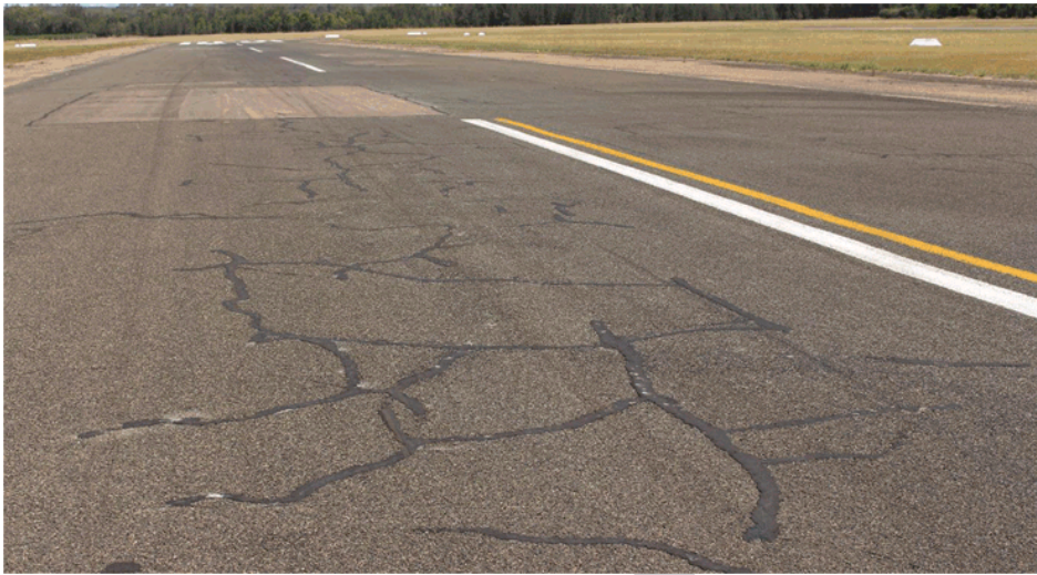
Figure 2-6 Excessive cracking and pumping east of runway centreline
