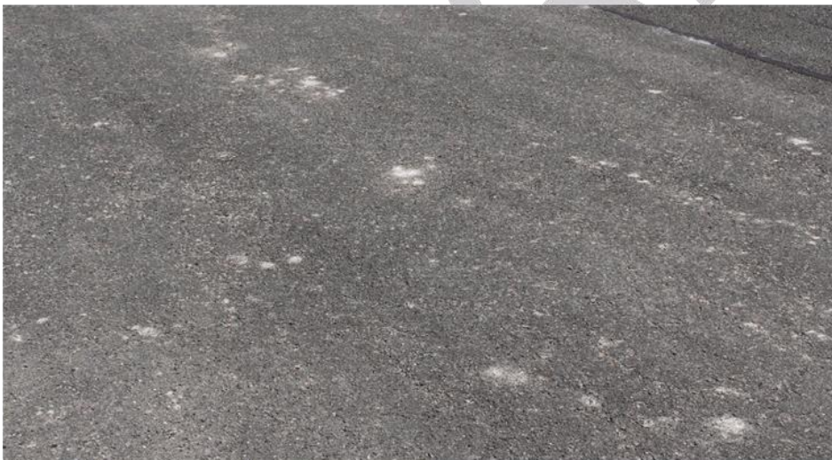
Figure 2-5 Pumping of material through wearing course
