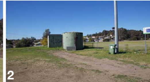
2 Existing water tank and storage container.
