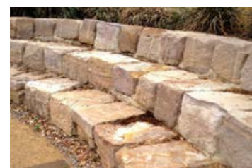
Stone and block work terracing
