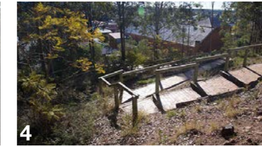
4 Existing stairs and handrails to CBD.
