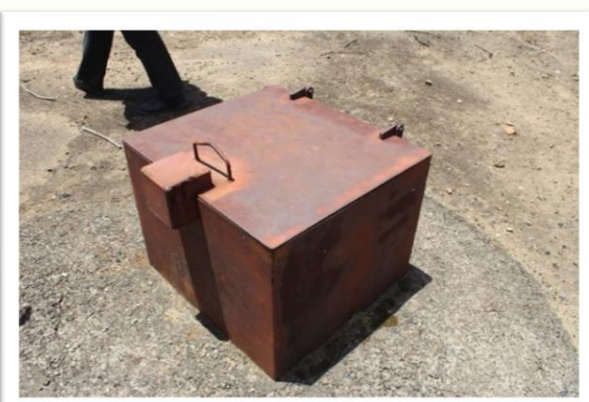
Figure 18: Second mine shaft cover
