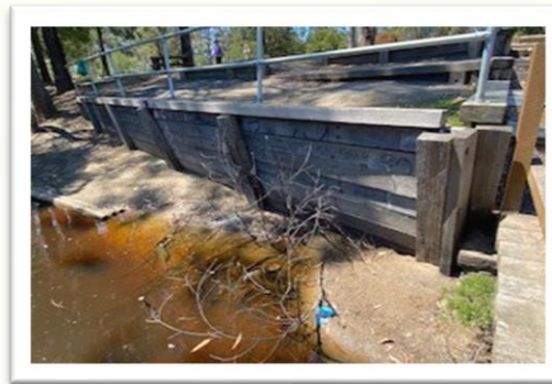
Figure 28: Viewing platform and retaining wall
