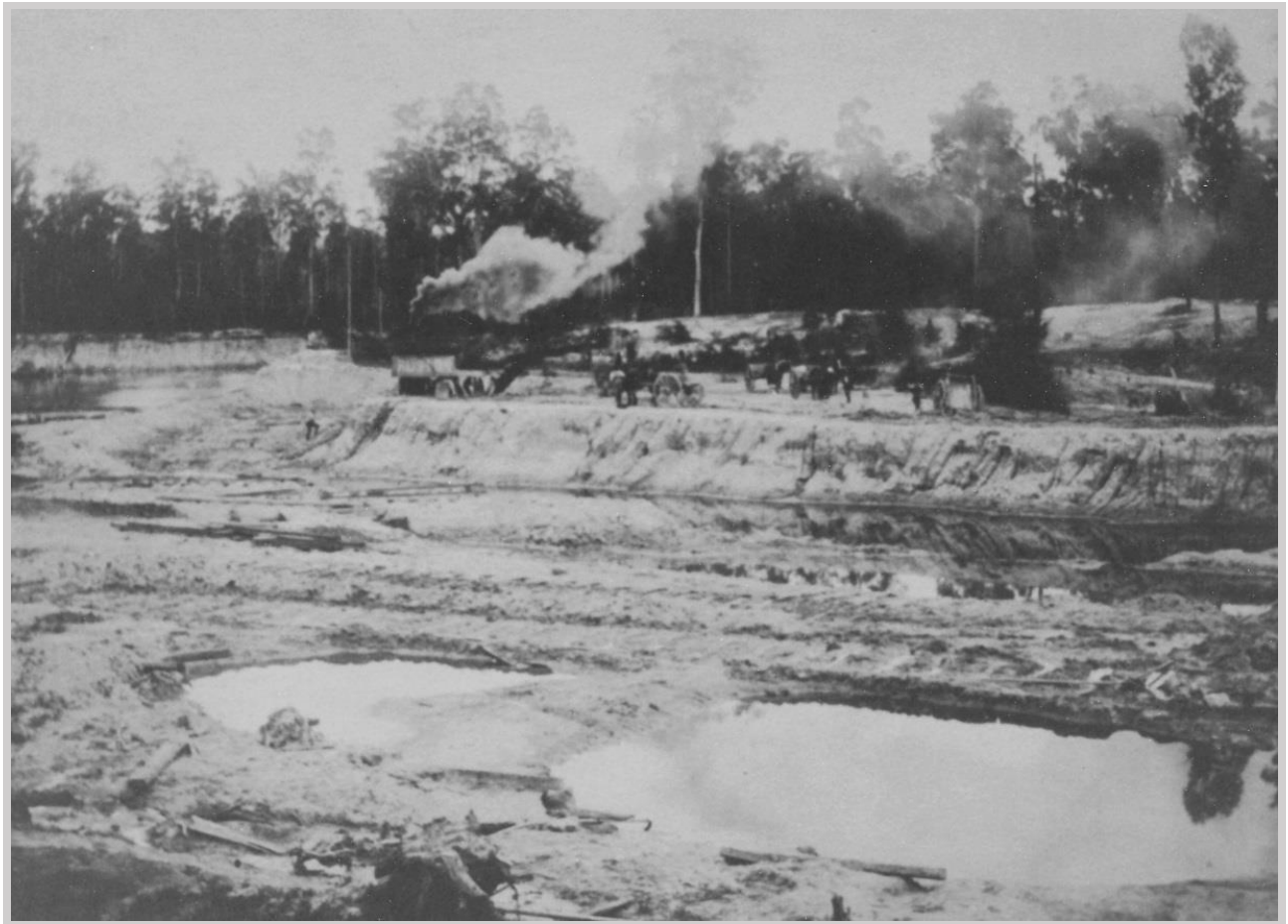
Figure 6: Photograph of the construction of the dam at Aberdare Central Colliery (Source: Newcastle Cultural Collections, Barry Howard Collection, accessed via Flickr).
