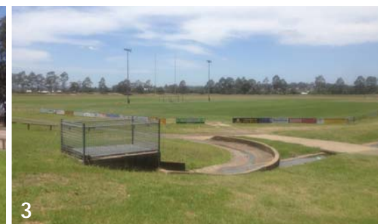
3 stormwater discharge - access constraint
