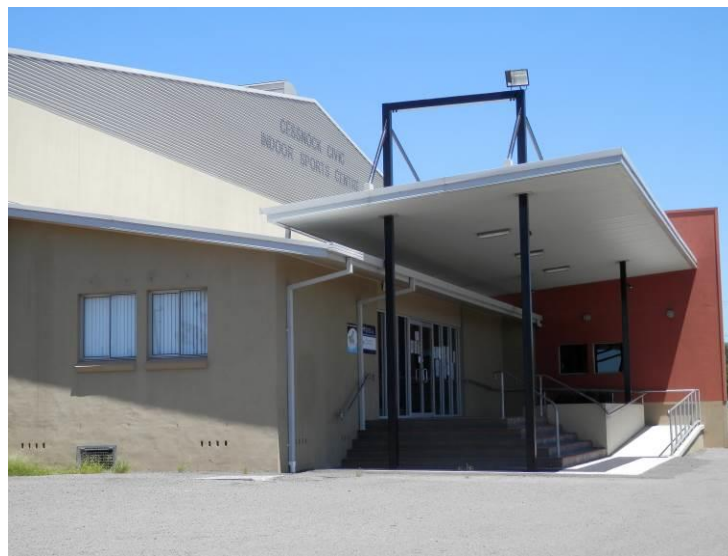
Above: Exterior of Cessnock Civic Indoor Sports Centre
