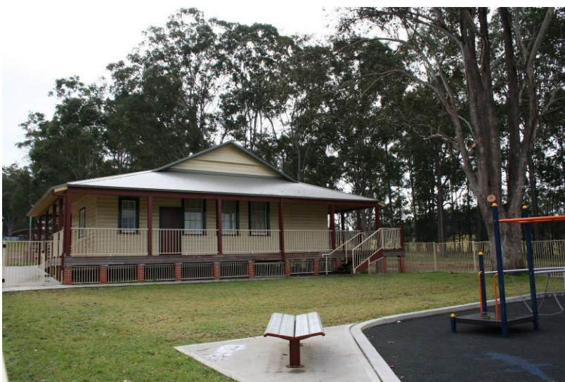
Left: Millfield Crawfordville Hall and surrounding precinct.
