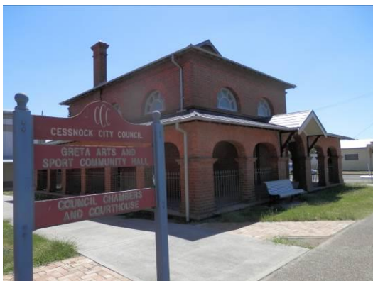
Above: Former Greta Courthouse, Fronts onto the New England Highway
